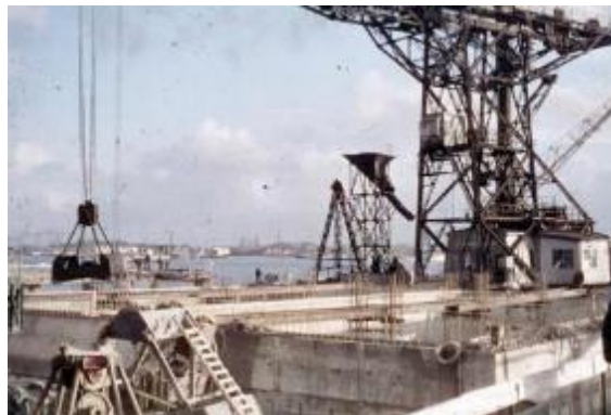
Figure 1: Bridges constructed in the 60s are still heavily used today [Beeldbank1]
