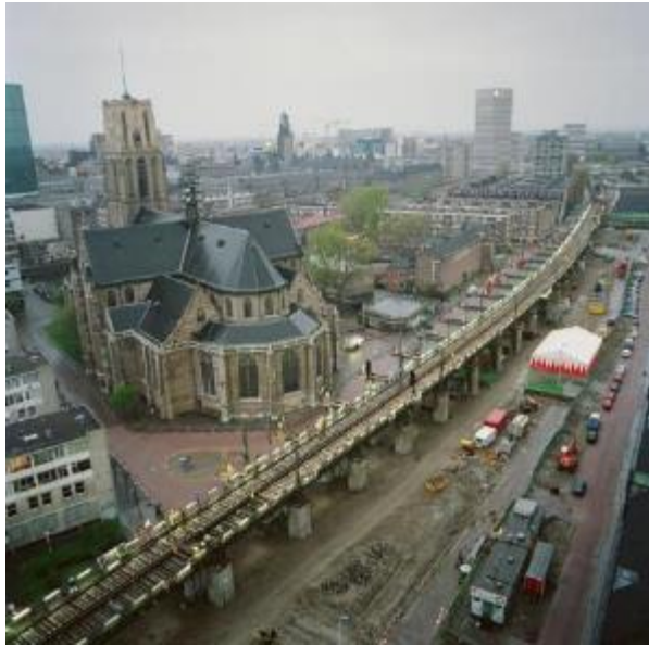
Figure 3: Limited space for infrastructure renewal (source: [Beeldbank2])
