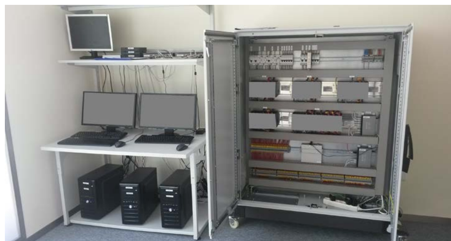
Figure 3: SCADA real equipment
